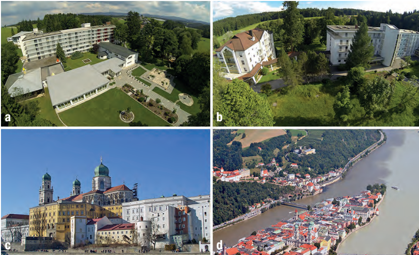
Fig. 1.85 Prof. Schedel Rehabilitation Center in Kellberg, near Passau (a, b). City of Passau (c). Aerial photograph of the city of Passau, where the Danube river is joined by the Inn and Ilz (d).
